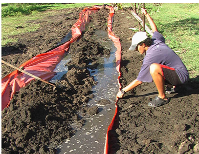
The trench can be filled with water to help adjust the level of the edge of the polythene so the water uniformly wicks into the plant bed.
