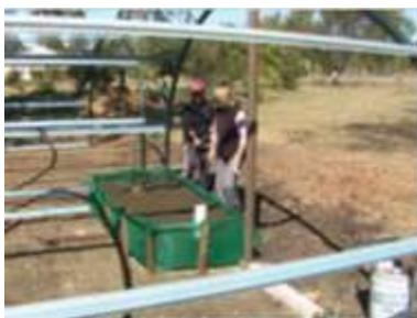
The reservoir is then formed by placing the polythene sheet in the base, laying in the pipe work, filling the reservoir with wood chips, then filling the root area with soil.
