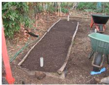
The simplest way of making a closed bed is to scoop out the top 200 or 300mm of soil, line the trench with plastics, place the distribution pipes, back fill with open organic mix and then replace the top soil to form a semi raised bed.
